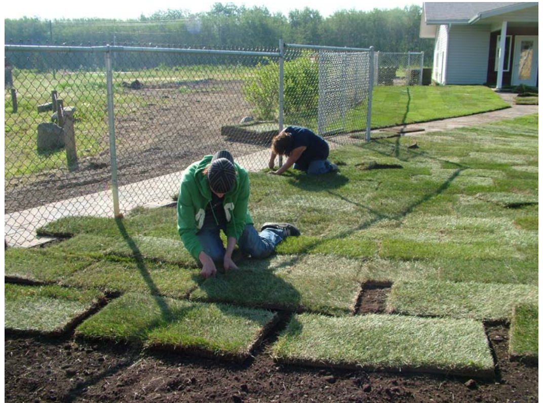
Sod being Placed at the Cree-Ative Playground by the local Youth hired by a Subcontractor
