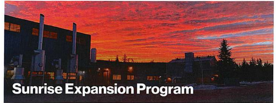
Image above: existing compressor station 5 – "Australian" – near Quesnel, BC
