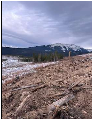
Figure 3. A recently recontoured road.
